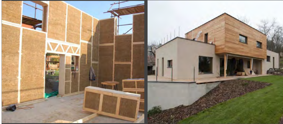
Panelized Straw Walls – EcoCocon – Lithuania - Bjorn Kiefulf, Architect
