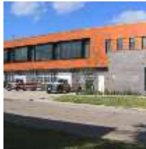
Johnson County Ambulance Center
