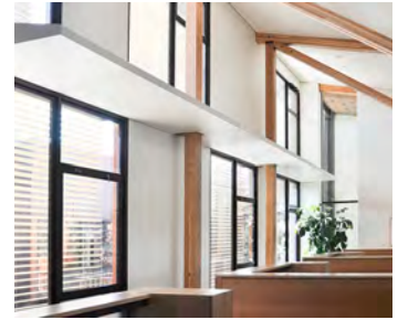
(Above) Interior light shelves to improve daylight penetration in exterior office spaces.
