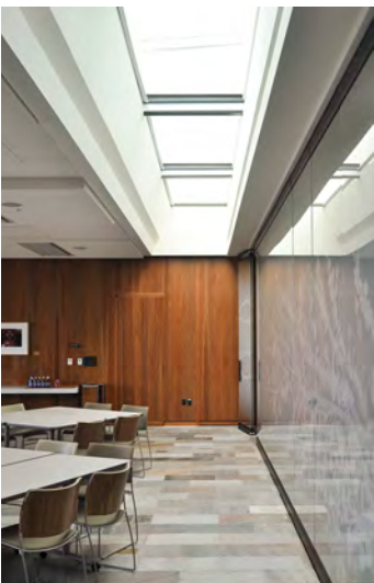
(Below) Daylighting via skylights at interior conference room. (Opposite page) Automatically operating exterior blinds on west-facing facade.
