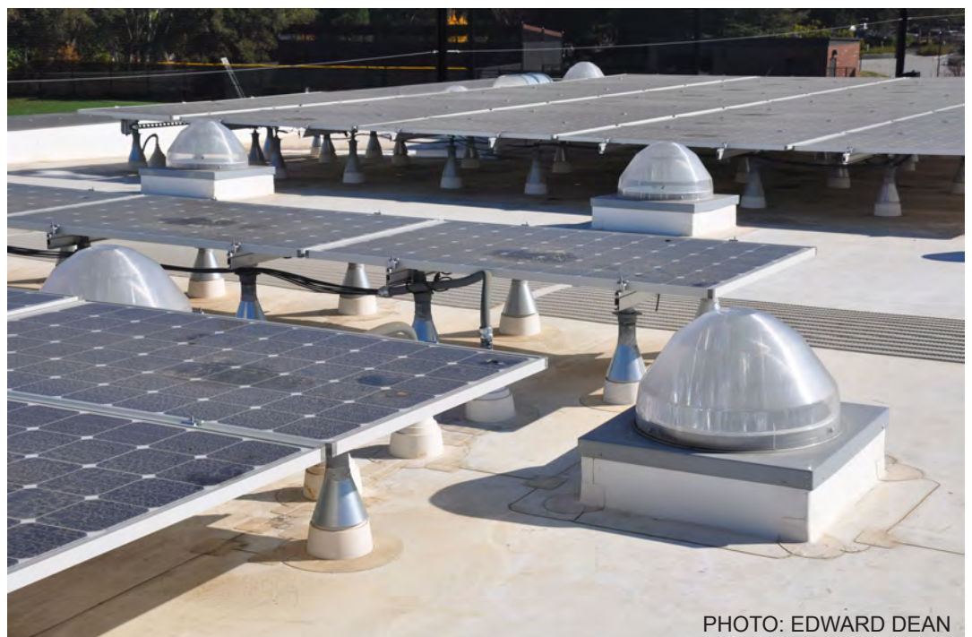
(Right) View of portion of roofscape consisting of solar photovoltaic panels laid flat and tubular skylights.
