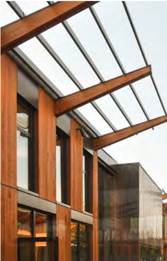
(Above) Overhang design for east-facing facade, allowing maximum daylight penetration while protecting against direct sun.
