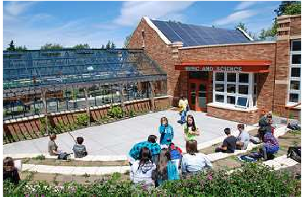
Hood River School District Science Building | Hood River, OR Photo Courtesy of Opsis Architecture
