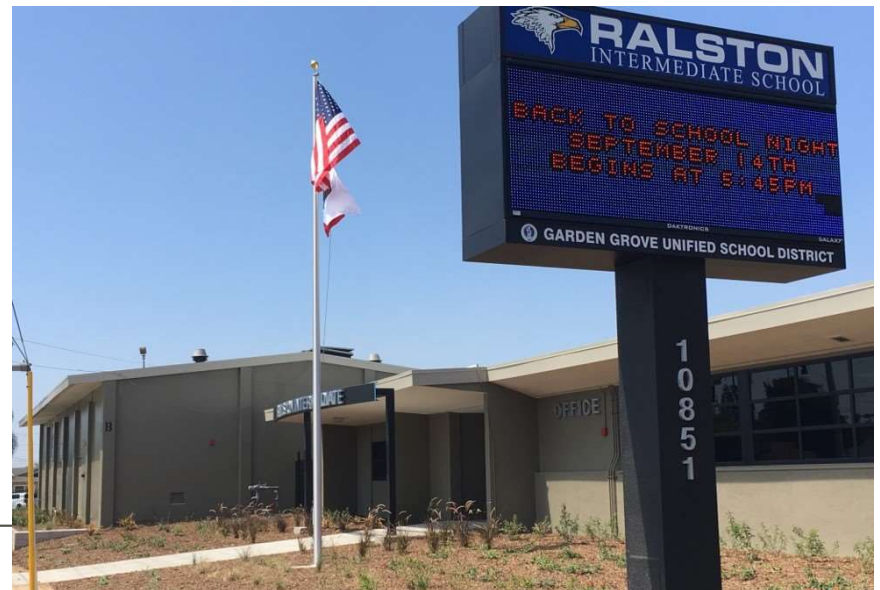
Photo Courtesy of Garden Grove School District.
