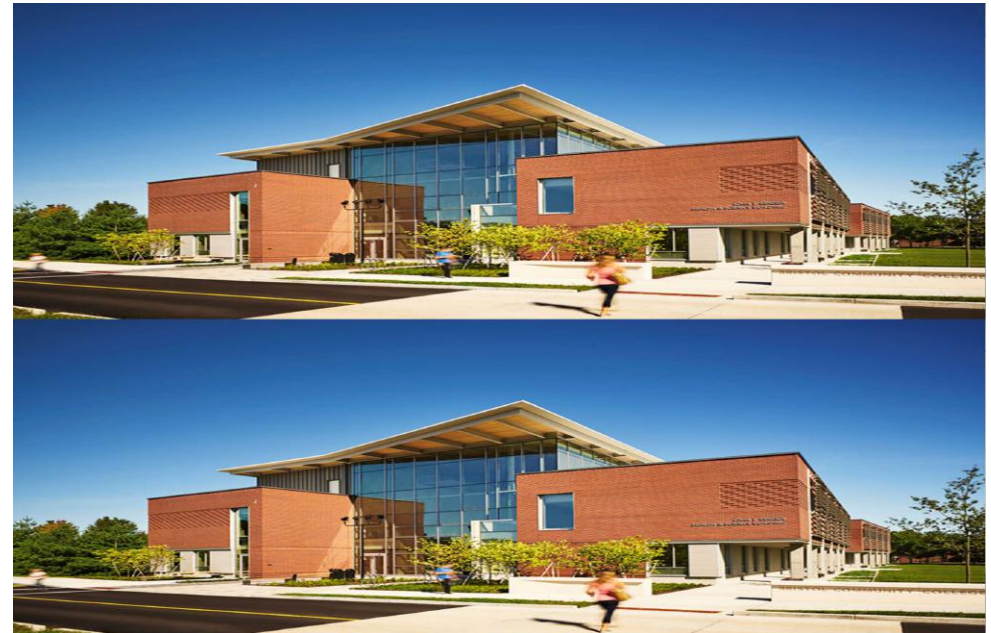
Sbrega Health & Science Building | Fall River, MA Photo Courtesy of Edward Caruso
