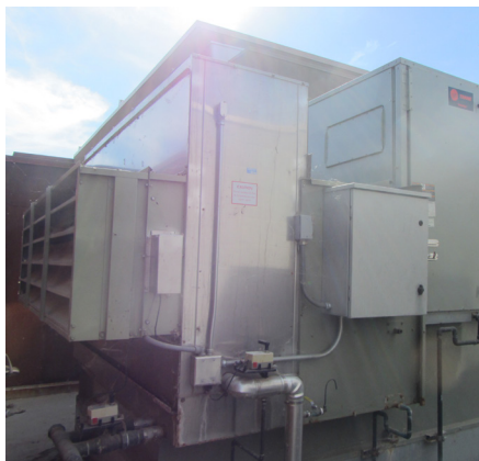
The Indirect Evaporative Cooling system at San Luis Wildlife Refuge Visitors Center (Source: U.S. Fish and Wildlife Service)
